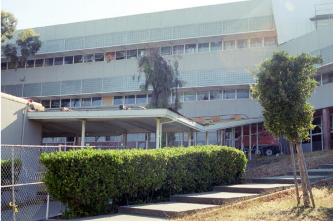
Figure 5: Rear of Main Classroom Building
