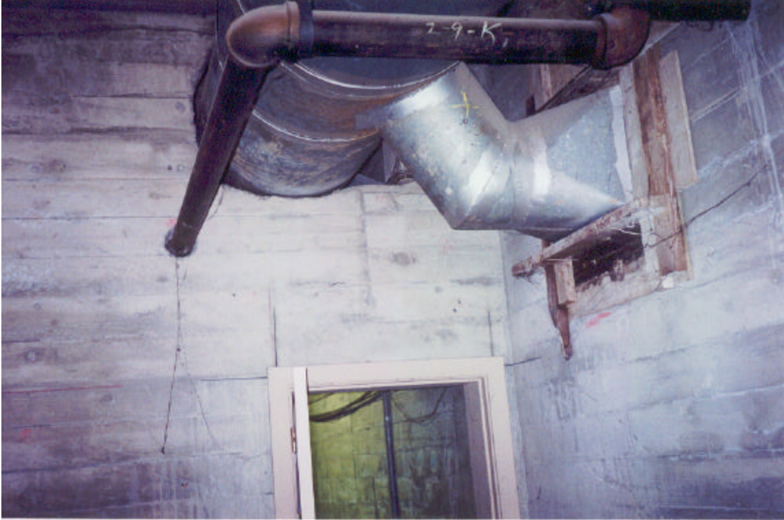
Figure 9: Sawcut opening in basement wall of Main Classroom Building
