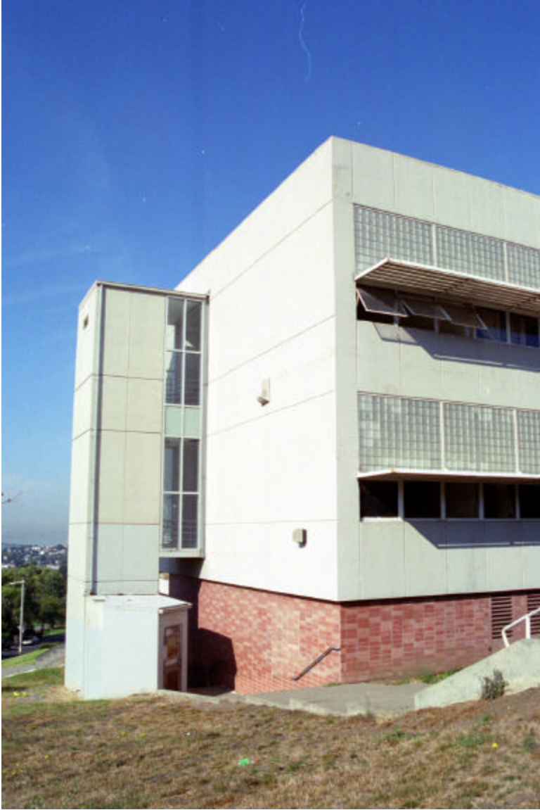
Figure 8: Elevator tower Main Classroom Building
