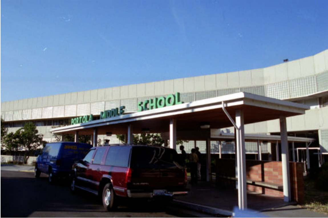
Figure 2: Front of Main Classroom Building
