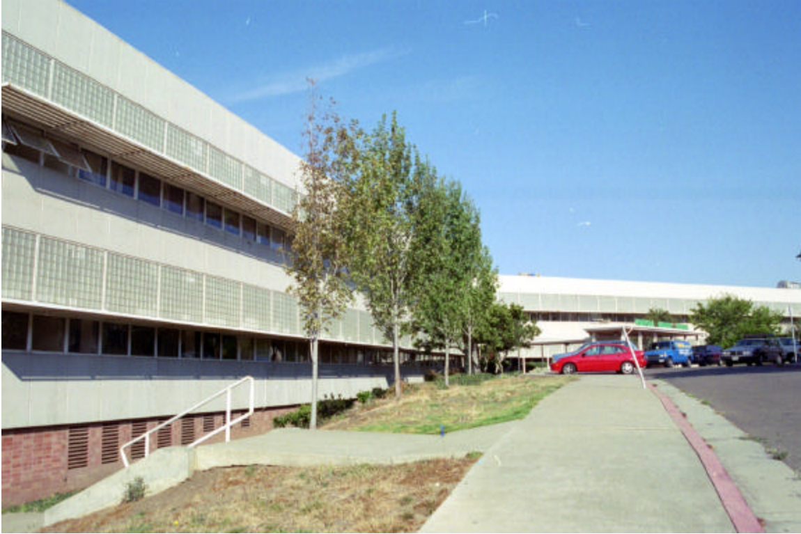
Figure 4: Front of Main Classroom Building
