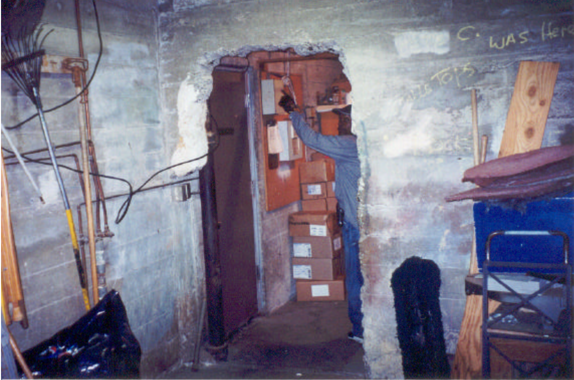
Figure 10: Rough cut opening in basement wall of Main Classroom Building
