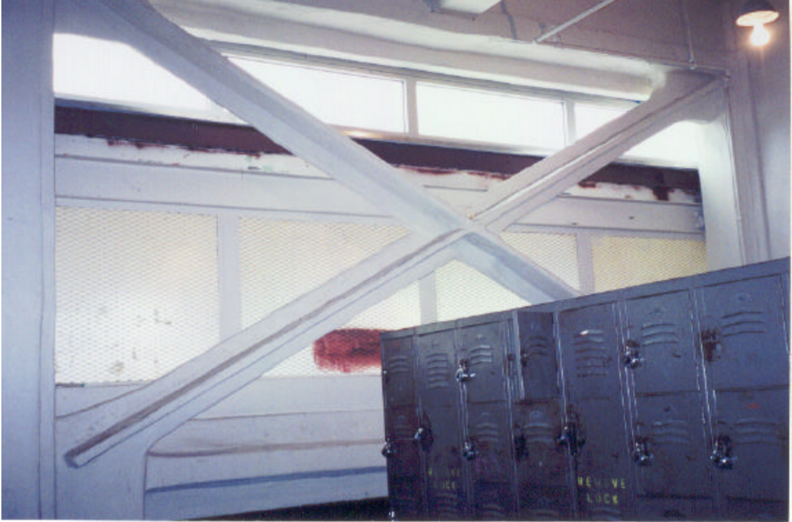
Figure 17: Retrofit bracing at interior of locker room
