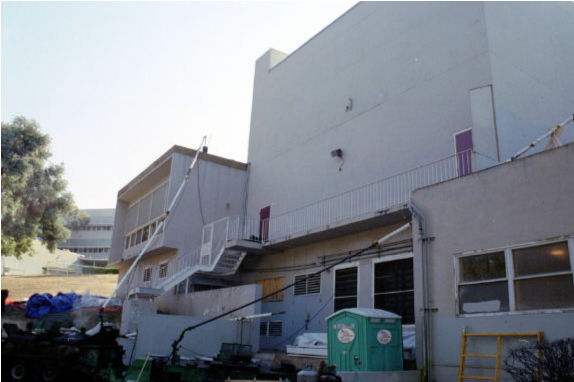
Figure 15: West side of Gymnasium Building
