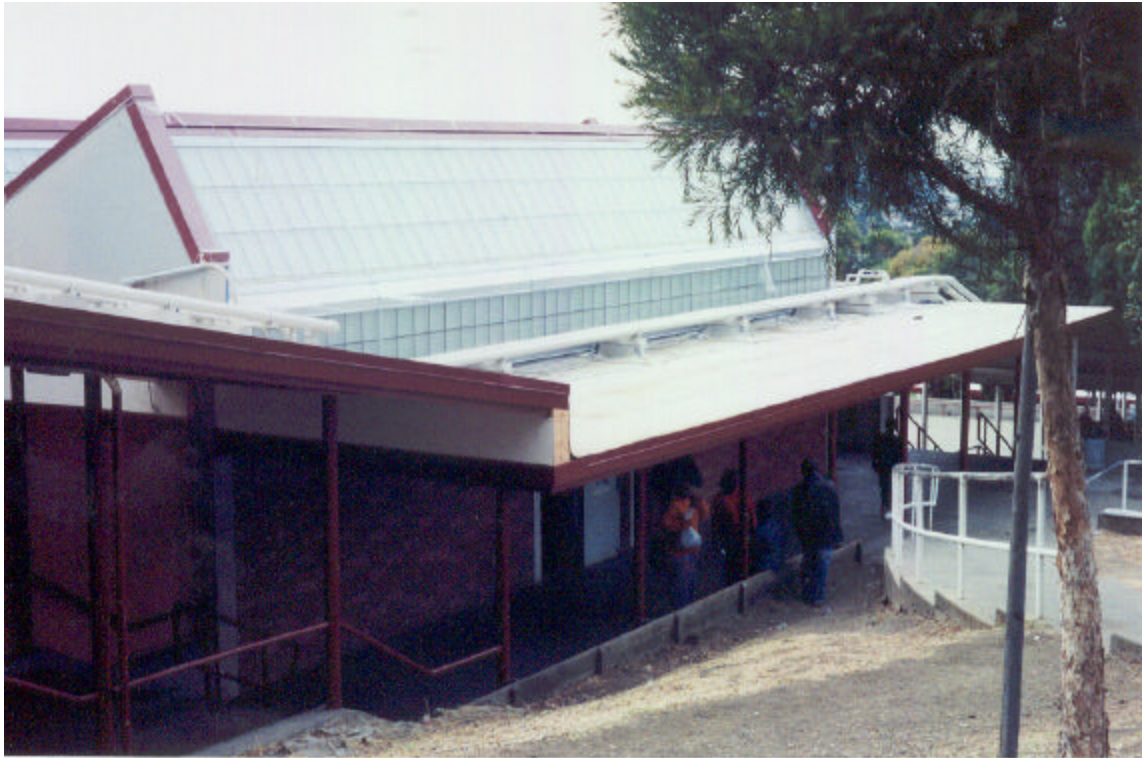
Figure 22: West view of Laboratory Building
