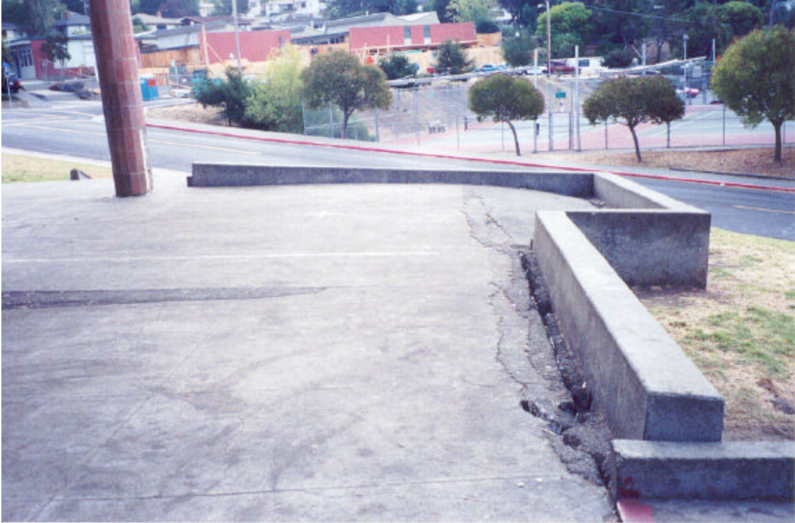
Figure 3: Settlement of site paving adjacent to Main Classroom Building
