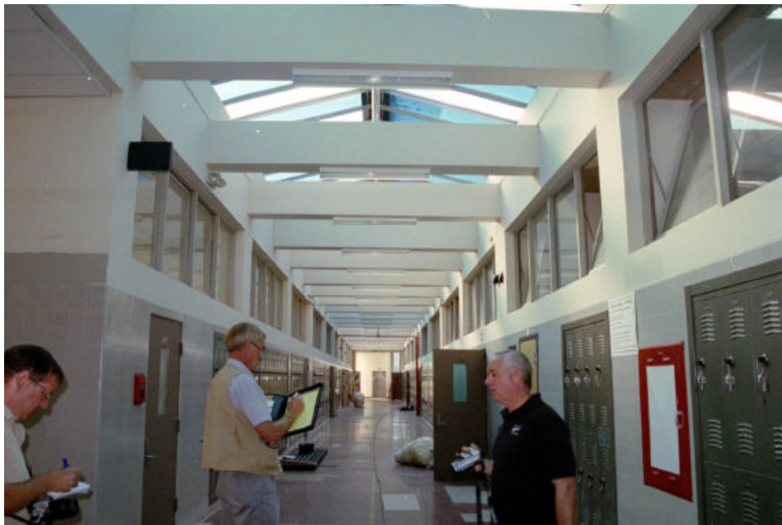
Figure 12: Central second floor corridor and skylights at Main Classroom Building
