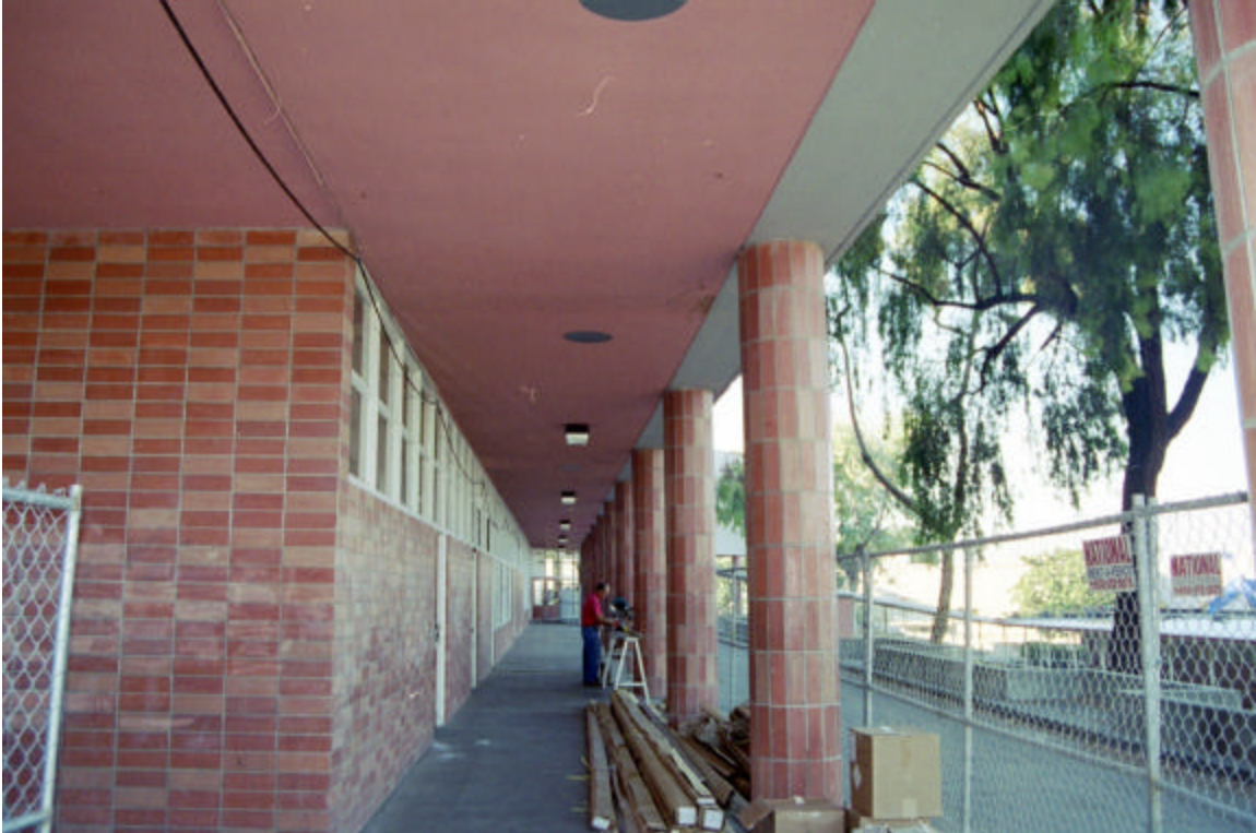
Figure 7: West side of Main Classroom Building at the ground floor
