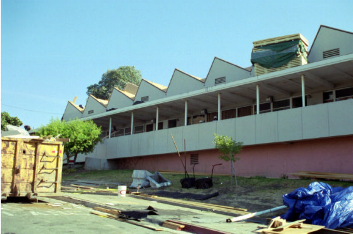
Figure 21: South view of Laboratory Building
