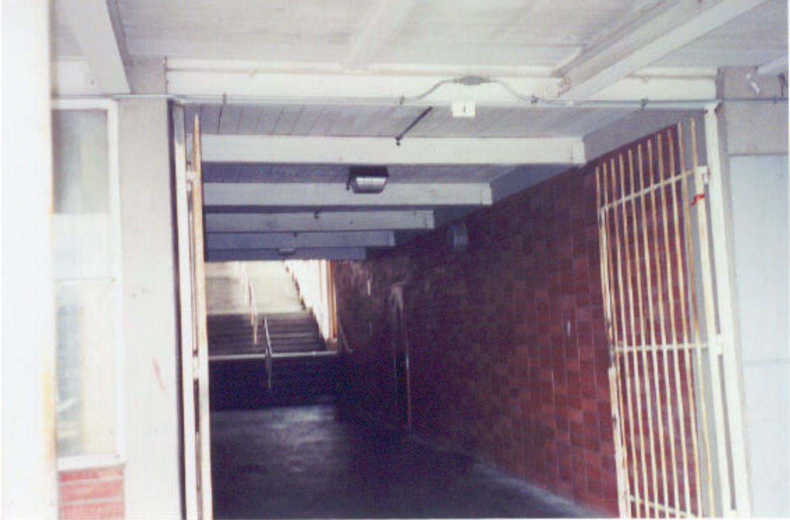
Figure 20: Covered walkway at Gymnasium Building between locker rooms and attached classroom building
