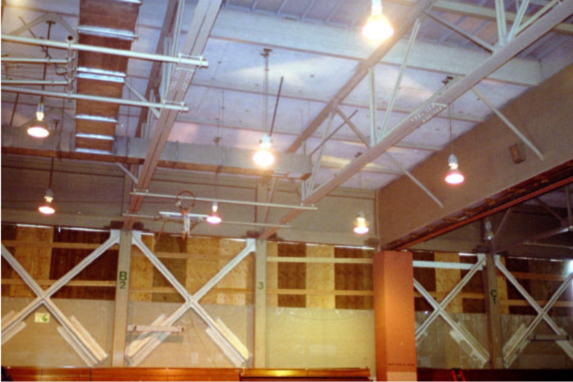
Figure 16: Retrofit bracing at interior of Gymnasium
