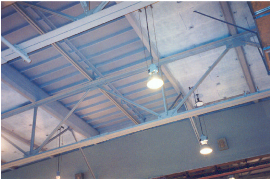
Figure 19: Infill of skylight openings at Gymnasium
