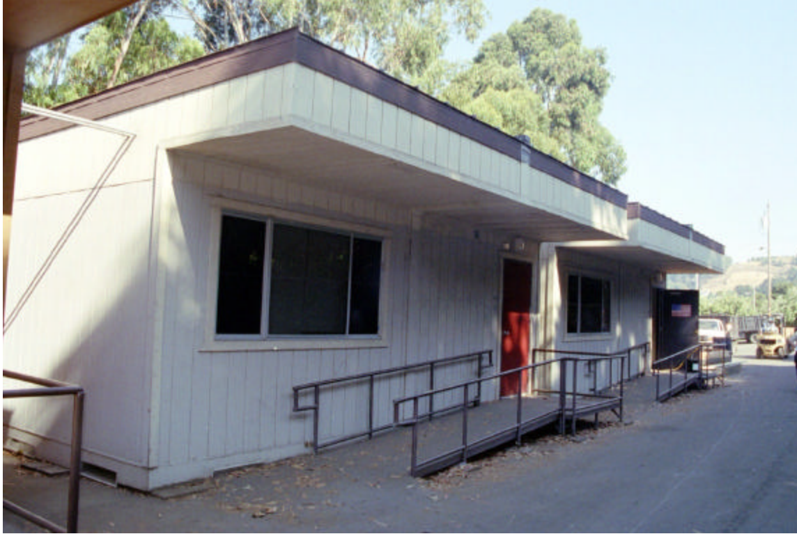
Figure 26: Conduit between portable classrooms
