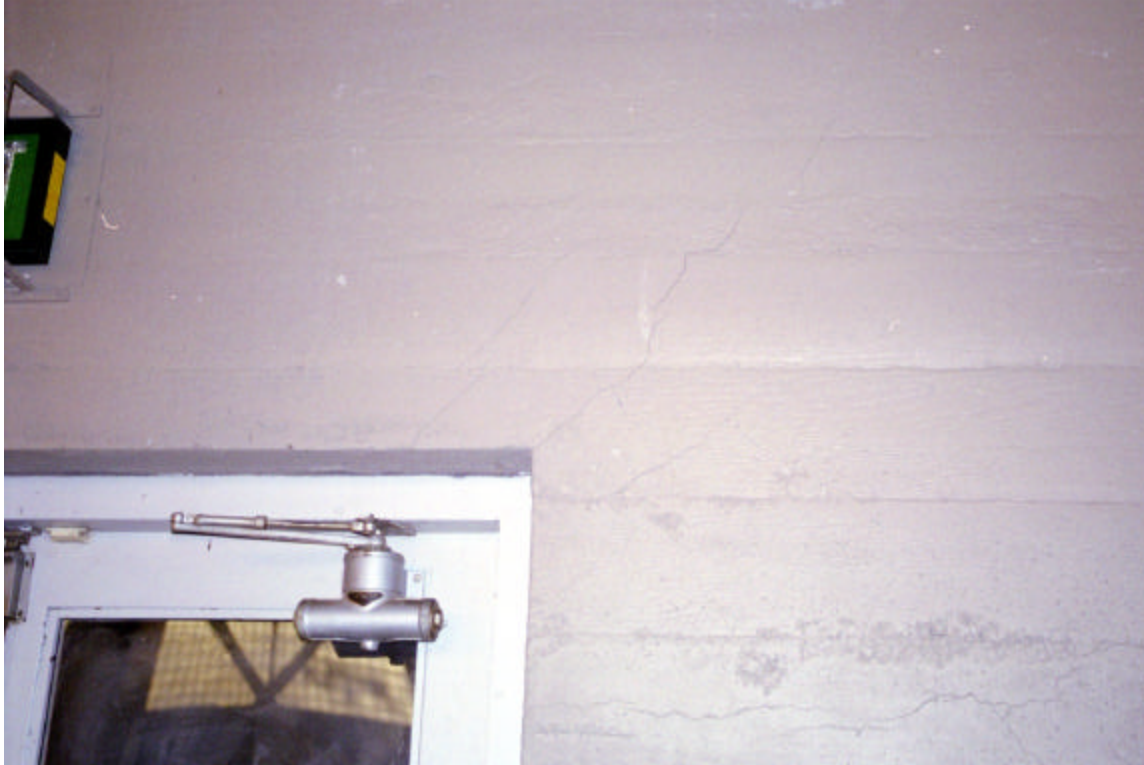
Figure 18: Cracks in the wall of Gymnasium Building
