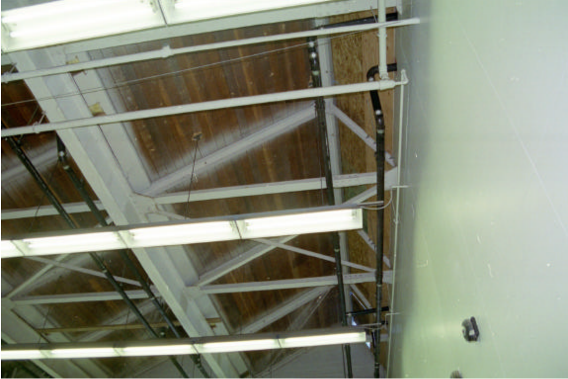
Figure 24: Sawtooth roof trusses at Laboratory Building
