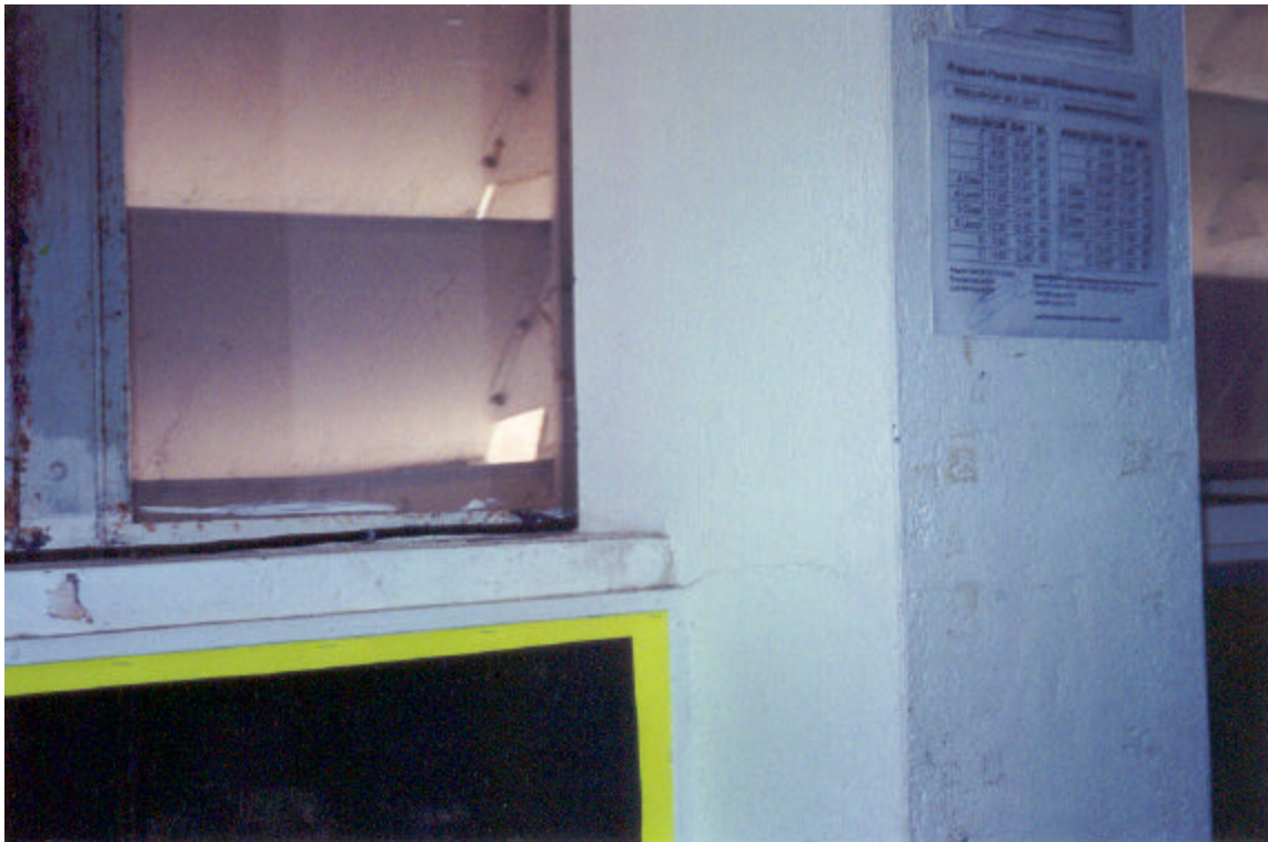
Figure 23: Cracks at the base of columns in Laboratory Building
