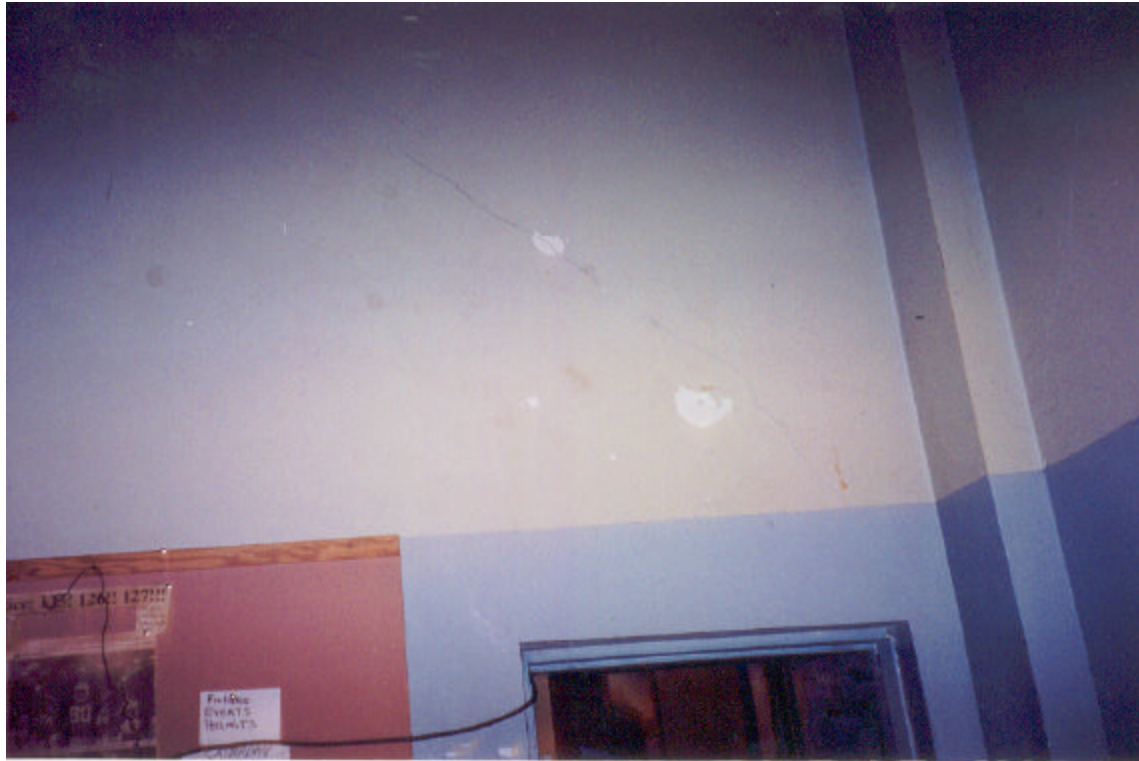
Figure 11: Diagonal cracking in the basement wall of Main Classroom Building
